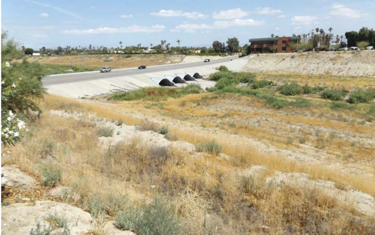
Photo 5: View to the north/northwest towards Cook Street from the CVWD access road along the southern levee of the stormwater channel
