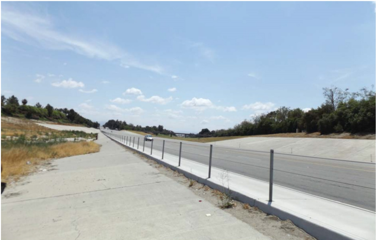
Photo 8: View to the east along Fred Waring Drive, from the southeastern portion of the channel, where it is traversed by the road
