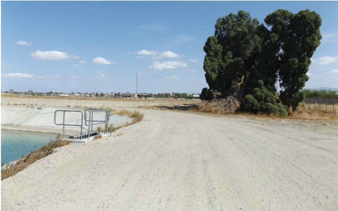
Photo 1: View from within the WRP10 site, along the eastern border, looking to the north towards the existing operational parking area
