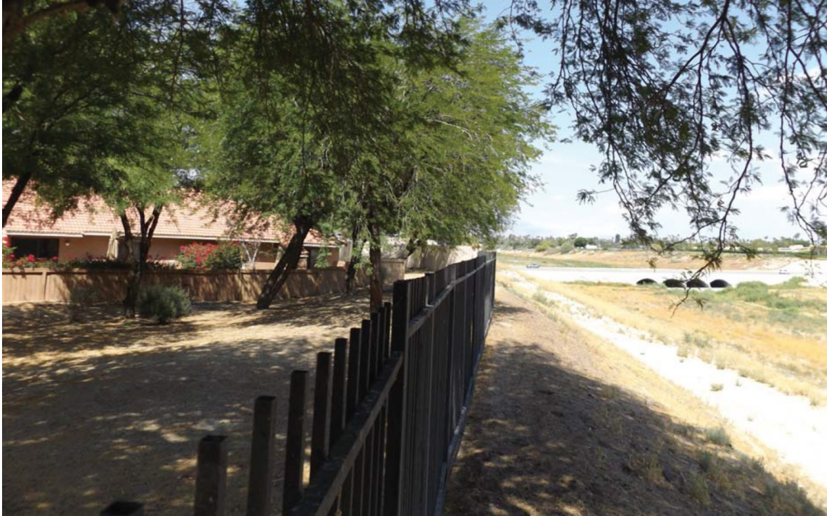
Photo 7: View to the west from the CVWD access road on the southern levee of the stormwater channel - backyards of residences in Palm Lake on the left
