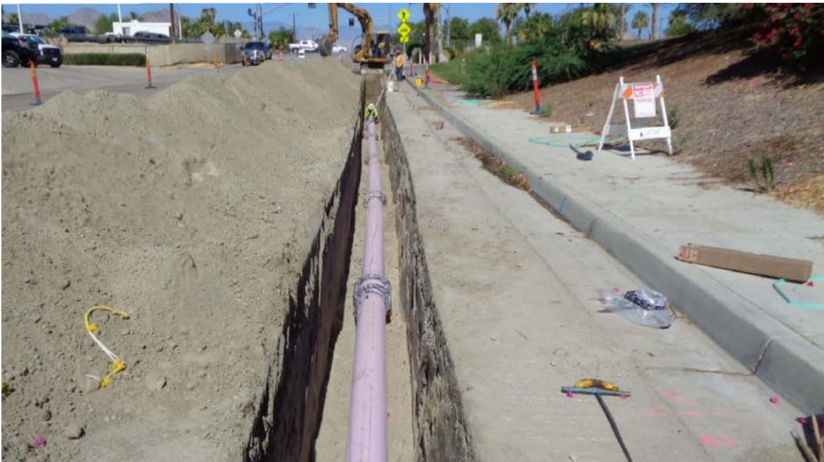
Figure 5 Typical Non-Potable Pipeline Trenching Work Site
