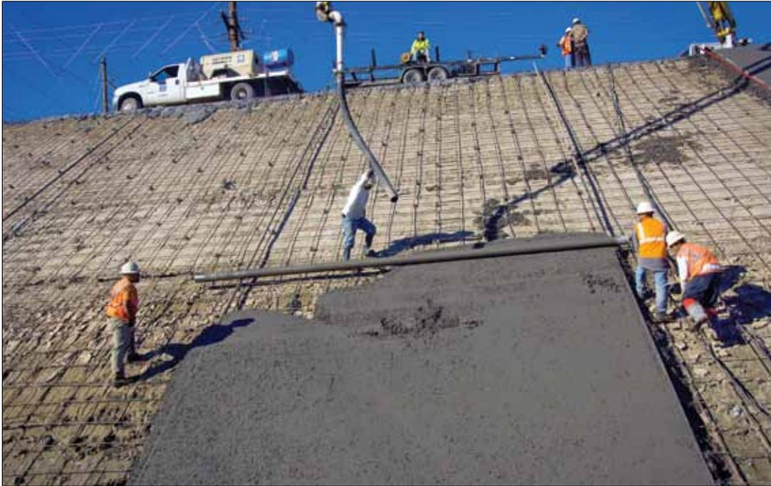
The Whitewater River and Coachella Valley stormwater channels convey flood waters from rain and snow melt safely through the valley to the Salton Sea. Concrete lining, sometimes hidden underneath golf courses, landscaping or earthen material, helps prevent erosion and protect adjacent properties.
